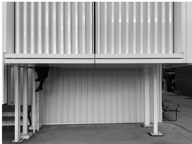
Scale 1: a mockup of the unitised façade
